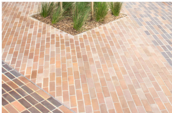
LOCALLY SOURCED CLAY BRICK PAVING
