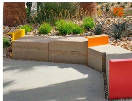
Cut local sandstone block seating
